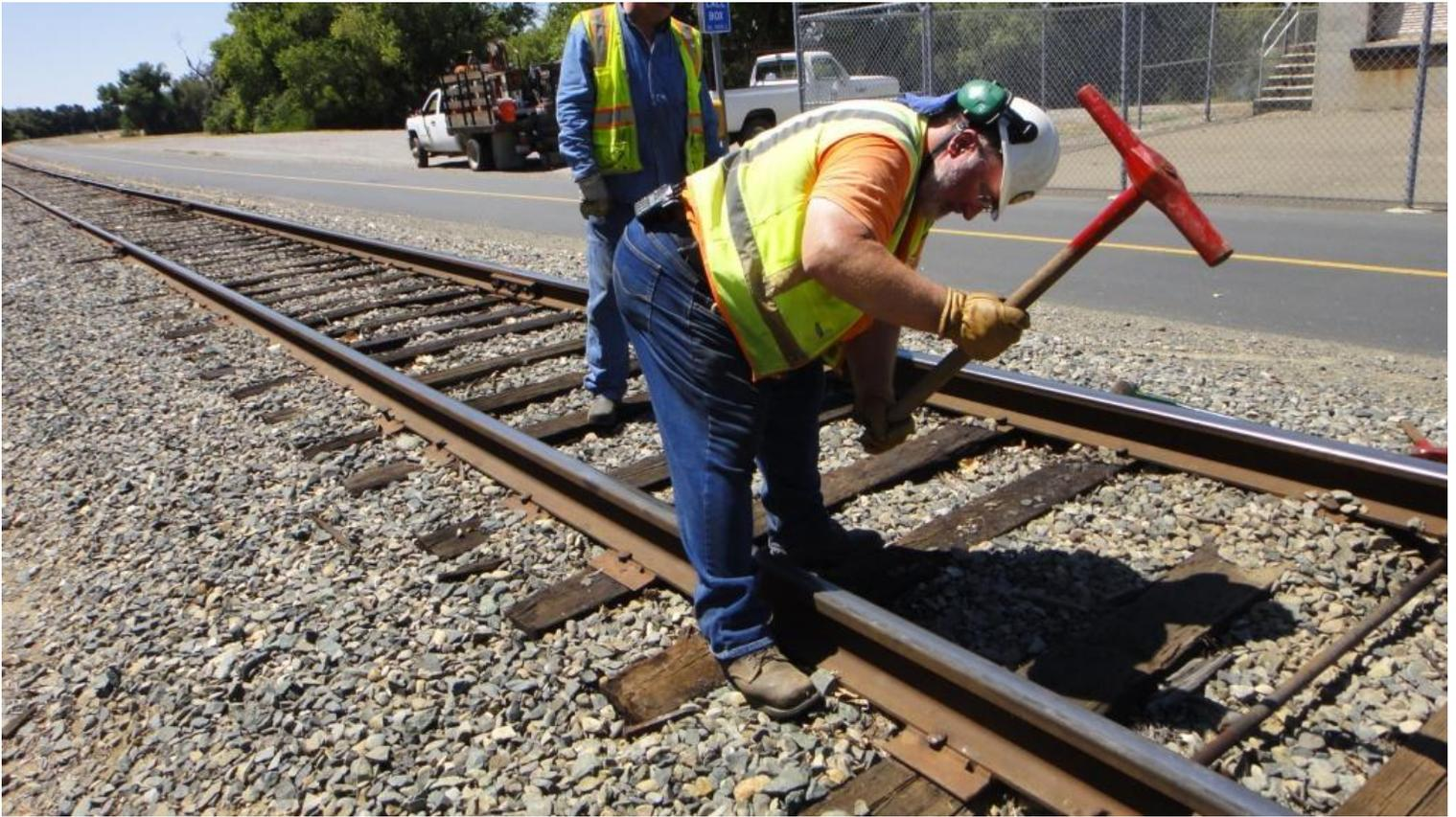
After the gauge-rods are tightened down Frank re-spike the re-gauged track
