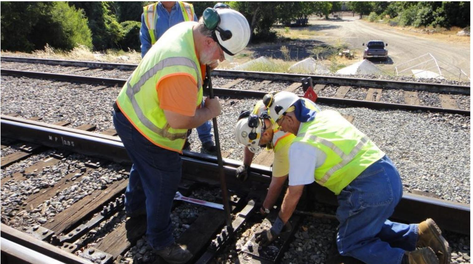
Meanwhile, at Switch 13 (South Clunie ground-throw), Frank uses a lining bar to make small adjustments to the connecting rod so that Mike F. and Clem can line up the bolt holes
